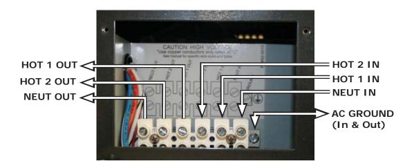
Figure 2-10, AC Terminal Block
